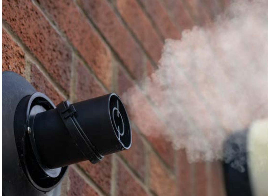
Plumbing from the flue showing a high temperature, inefficient boiler
