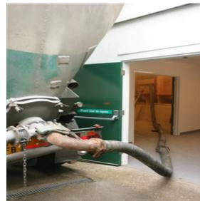
The boiler house needs to be adjacent to the fuel store because the screw feed system should not be too long (3m). There are systems on the market that can suck the pellets into a small hopper. These can cope with distances of 15m.
