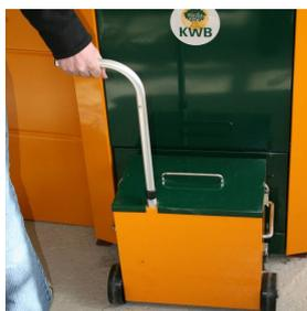
The ash may need to be removed up to once every three weeks depending on the model, fuel usage, type of fuel and time of year. Some models may only need to be emptied once every three months. The small amount of ash that is removed can be used as a high grade fertiliser.
