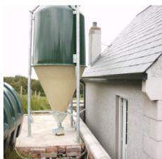
The floors of the silo should have a slope of at least 45° going towards the feed mechanism. A deflection mat should hang in the path of the pellets being blown into the storage unit.
